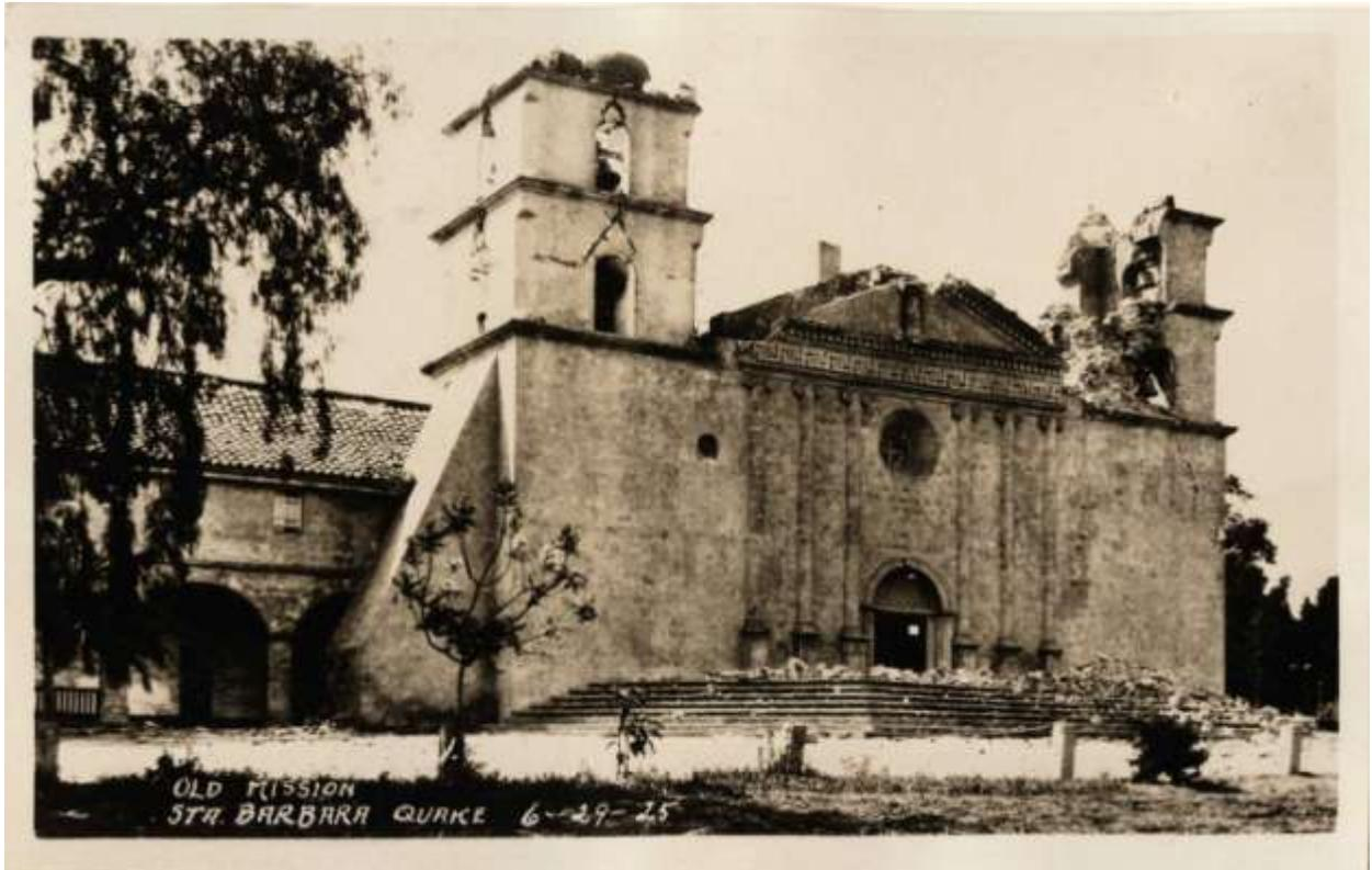
On June 29, 1925 a violent 6.8 earthquake on an early Sunday morning tore loose portions of the two bell towers, raining down large stones. One can only imagine what it must have been like to have been inside the chapel as the towers collapsed, for it occurred on a Sunday morning during Mass. The priest called out for the parishioners to stay where they were, perhaps saying a prayer, and when the
