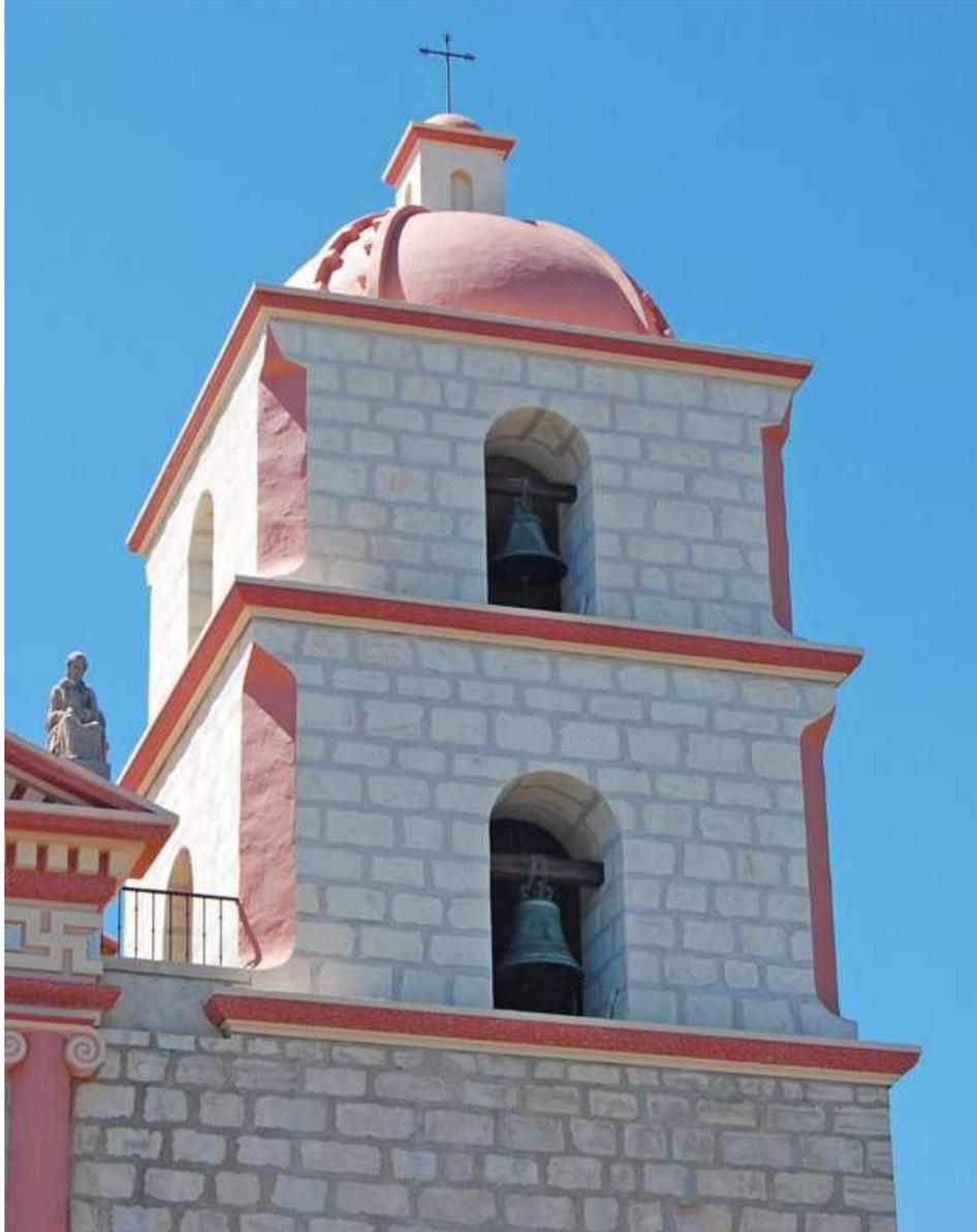
Look up at the bell towers and observe the difference between the stone façade and the painted stones on the towers after they were rebuilt with concrete and rebar so that
